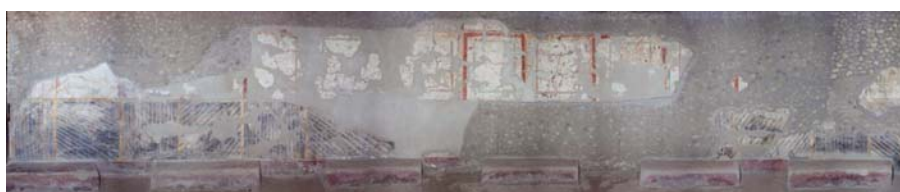
Abb. 3: Room 46, North wall
